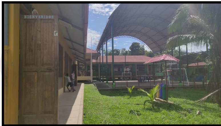
FIGURA 131: VISTA INTERIOR IE INICIAL 373 SHIVANKORENI
